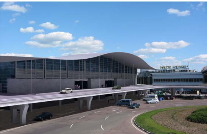
Kiev Airport. New Terminal Building. Ukraine.
